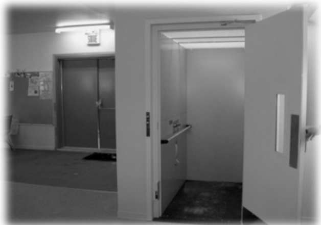
Open door leading to the new elevator.
